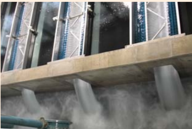
CH2M Hill "Prairie Waters Project Peter Binney Facility" Client: Aurora Water
